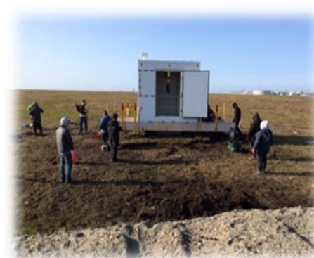
Foundation and local volunteers continue construction
